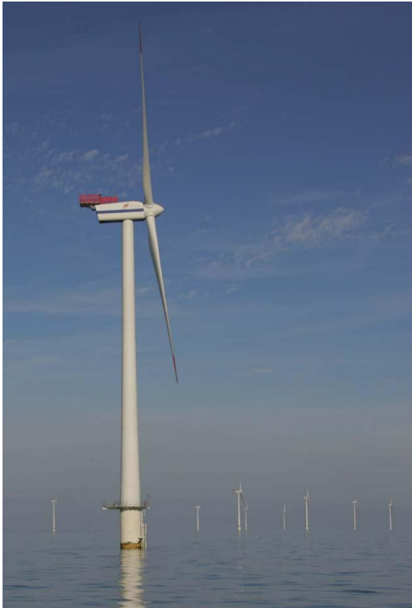
Turbine Vestas Horns Rev I
