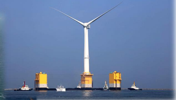
Mitsubishi 7MW oil pressure drive-type 2015
